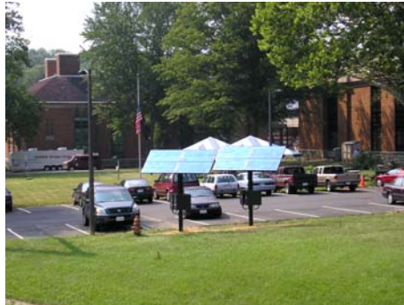
➤ POLE MOUNTED GROUND MOUNTED
